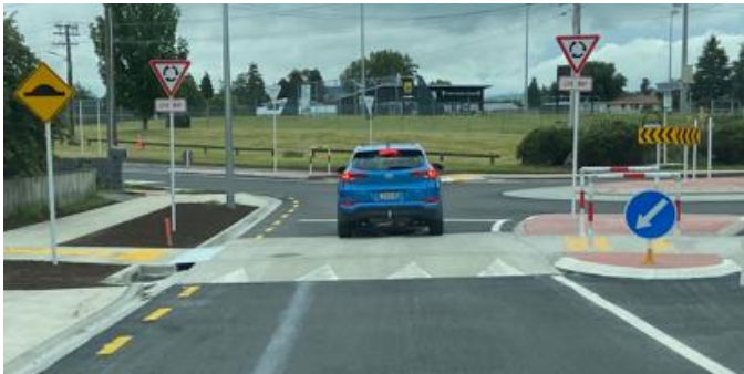
New roundabout providing effective flow of traffic at Taharepa/Tauhara Rds
