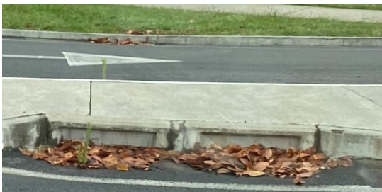
Detritus blocking drain sumps in urban area
