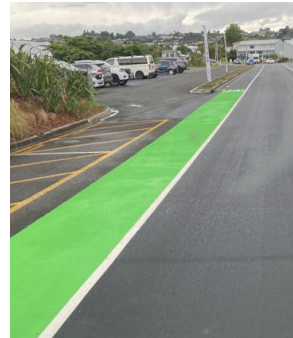
Example of cycle lane green paint work
