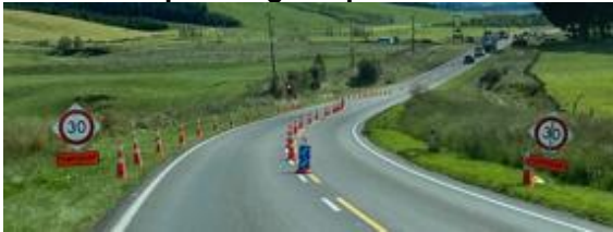
Example of good traffic management set up on Broadlands Rd
