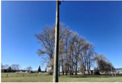
Existing timber light pole and fitting beside the playing field.
