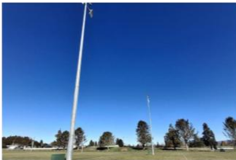
Existing metal lighting towers across the playing field.
