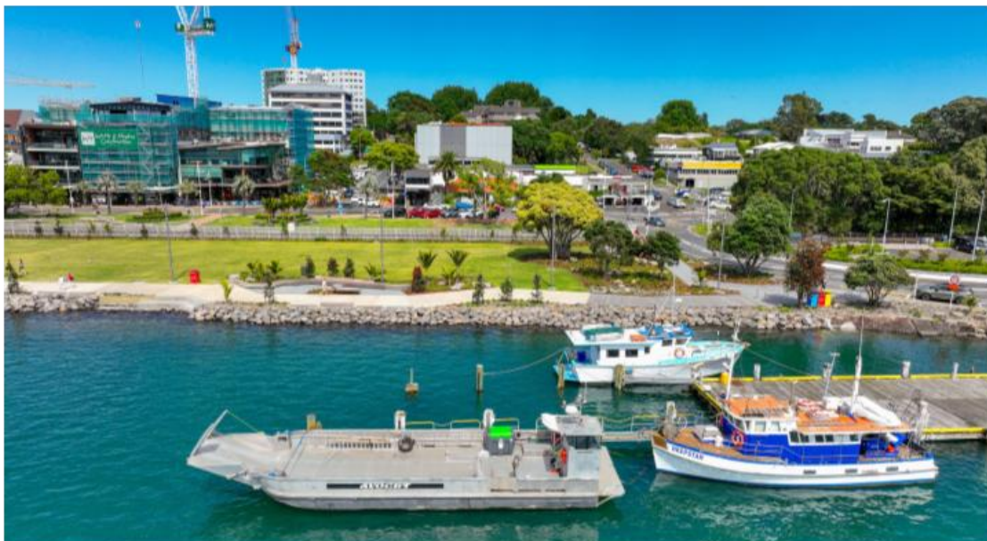
Upgrading of the seawall at The Strand, Tauranga City Council
