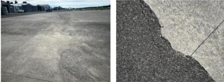
Figure 3-15: GA Apron: Concrete
