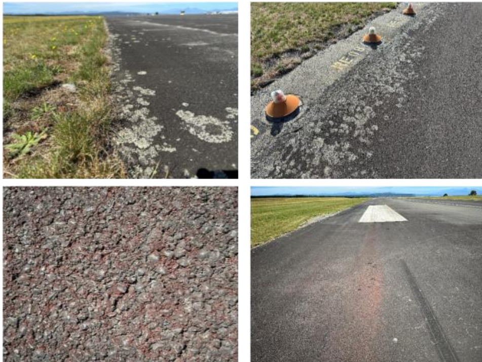
Figure 3-5: Main Runway – raised grass growth and red algae build up
